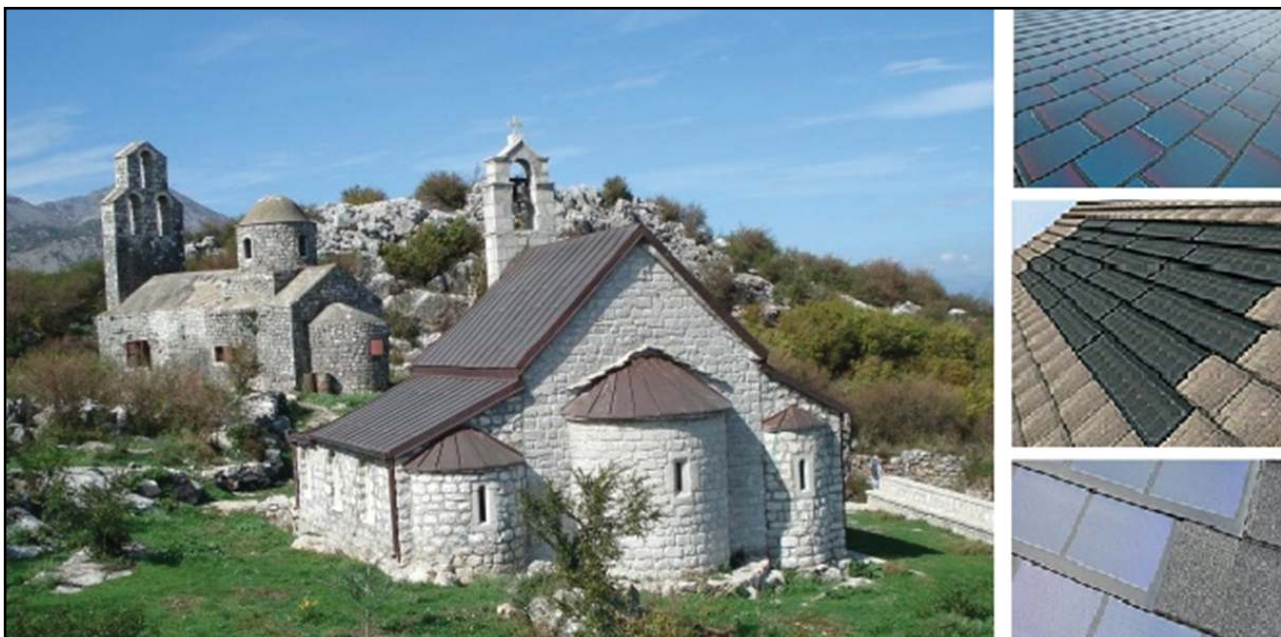
Figure 2: Building-integrated photovoltaics (BIPV). The Beska monastery, model
