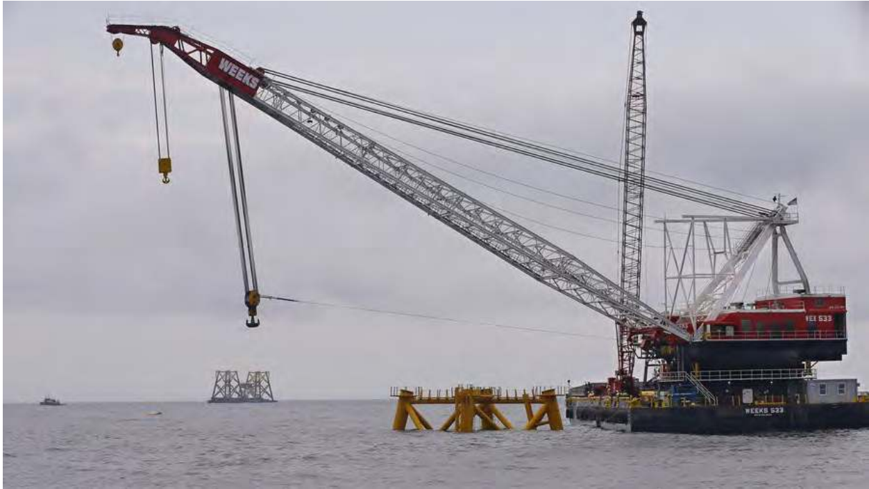
Figure 9. The 30-megawatt Block Island Wind Farm under construction. Photo courtesy of Deepwater Wind
