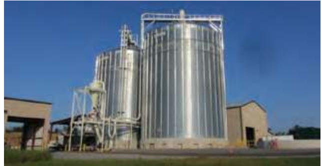
Figure 6.5 | In a project led by TennEra LLC, innovative technologies for (top) handling and (bottom) compacting forage harvester-chopped biomass increased bulk flow rates compared with tub-ground bales, resulting in reduced downstream processing and handling costs.
