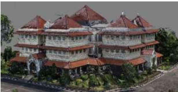
Figure 5. Dense Point Cloud of Library Building from aerial and terrestrial Photogrammetry
