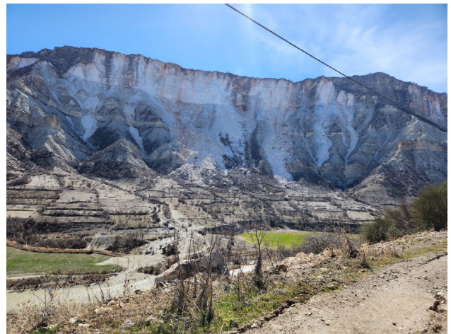
Figure 19. A view from the rock avalanches along the east slopes of the Göksu river
