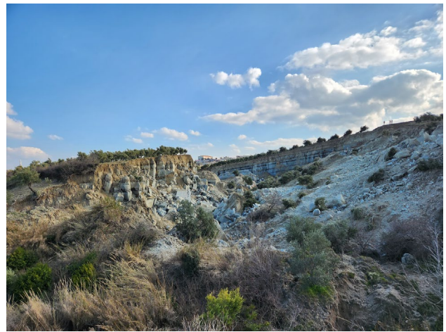
Figure 13. A view from the Tepehan planar failure triggered by the earthquake
