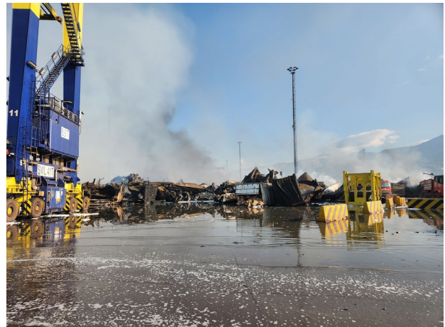
Figure 23. A view from the İskenderun Port after the earthquake
