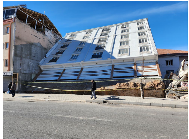
Figure 22. A toppled building due to liquefaction in Gölbaşı
