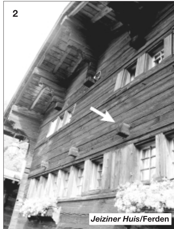
Photos 1, 2: Comparison of the Bach Huis (AD 1502, tree-ring dated) with a ridge-transverse main room beam (black arrow) and the Jeiziner Huis (AD 1591, by inscription) with ridge-parallel beams (white arrow). These construction techniques are representative for differing construction periods
