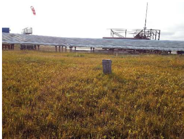
Figure E3. Location of the 2006 borehole (wooden box) showing the proximity of the new water supply system (a silver metal structure extending above the tundra surface since 2013).
