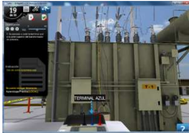
Fig. 2. Testing a transformer. The VR system shows step by step how to perform an electrical test. The trainee is supported by a control panel with several controls and instructions.
