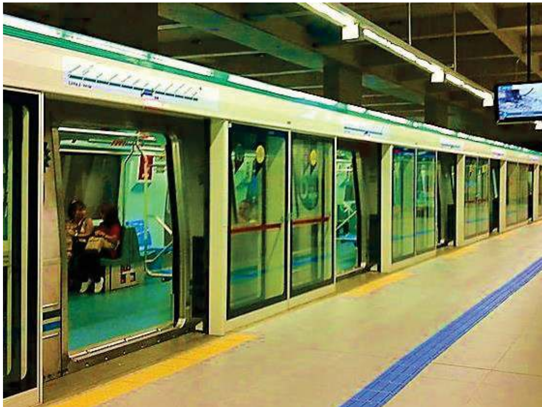
Figure 6.1: A platform screen door system installed at the Sao Paulo, Brazil
