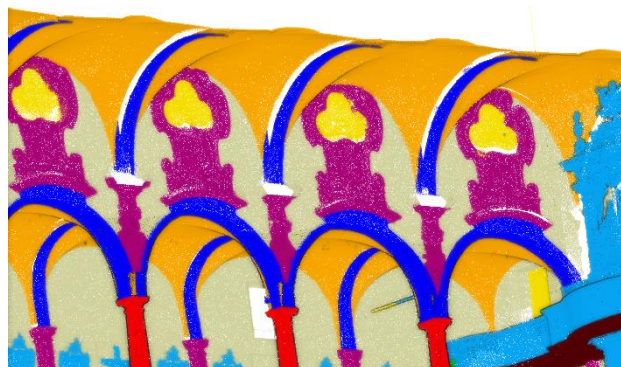
Figure 6. Examples of arches (blue) at a different height from the vaults (orange).
