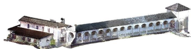
Figure 1. Point cloud of the portico of the Sacro Monte di Ghiffa (SMG).
