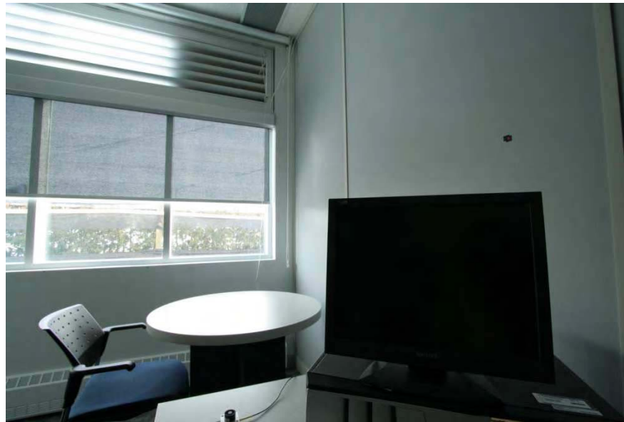
Figure 2 The two-element internal shading system was introduced for later trials in Room B, consisting of an upper Venetian blind with manual control, and a lower, motorized, opaque roller blind
