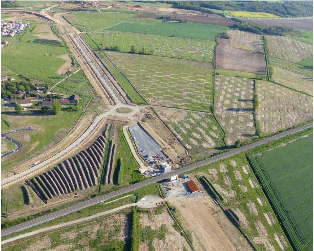
Aerial view of EIP area (west)
