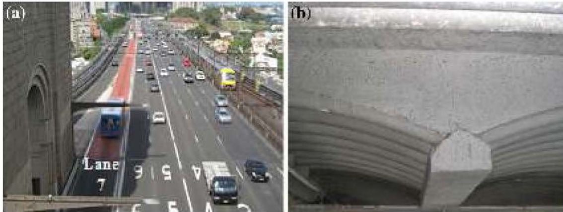
Fig. 2 Illustration of a the bus lane on the Sydney Harbour Bridge and b one of the concrete jack arches underneath the bus lane
