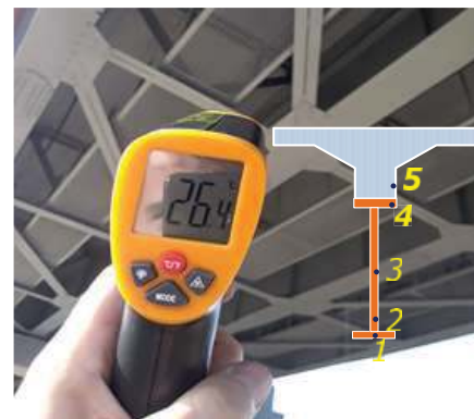
Fig. 2. Temperature measurement at the surface of the reinforced concrete beam of the bridge
