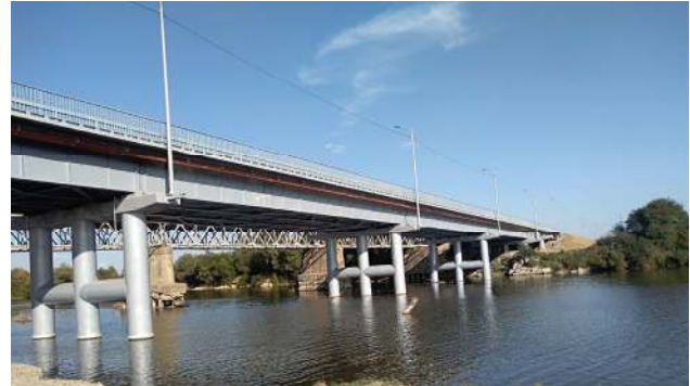
Fig. 1. Facade of the investigated bridge (Ukraine)
