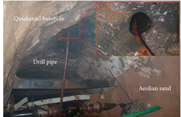
FIGURE 7: Borehole and chamber photo after quicksand disaster.
