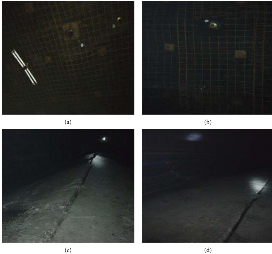
FIGURE 7: Deformation and failure of roadway-surrounding rock. (a) Roof. (b) Roadway side. (c) Floor. (d) Floor.
