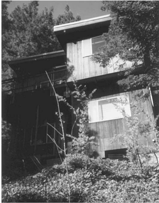
FIG. 11. A view of the country house hand-built by the Le Cams.
