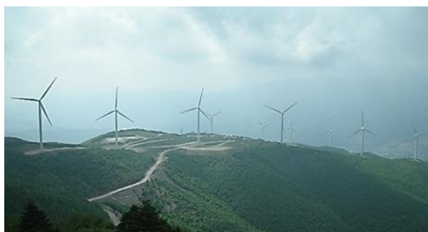
Figure 1. General view of the Belen Wind Farm.
