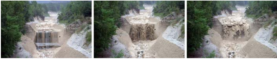
Fig. 3 Arrival of the debris-flow front upstream of check dam 29 during the July 28, 2006 event (C. Gwerder, WSL)
