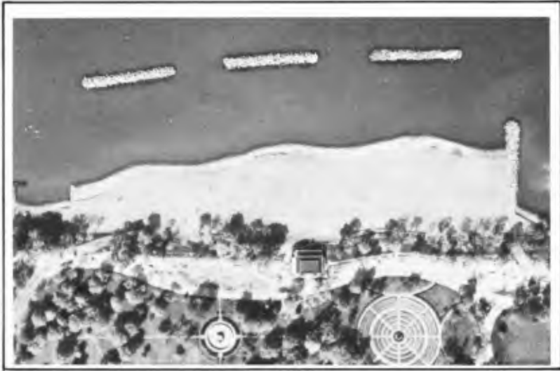
PHOTO 1: IMMEDIATELY AFTER CONSTRUCTION, OCTOBER, 1977
