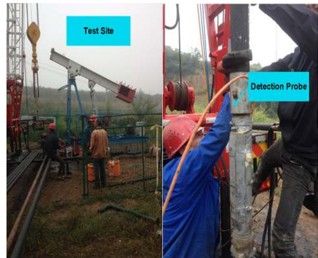
Fig. 8 Field photographs to show the detection probe entering a well
