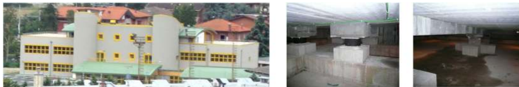
Figure 1. Left: the new seismically isolated primary school in Marzabotto (Bologna), former Italian seismic zone 3, which was opened to activity in September 2010, with safety certification of Dr. Martelli. At the center and right: two of the 28 high damping rubber bearings and one of the 14 sliding devices that form the seismic isolation system of the school.
