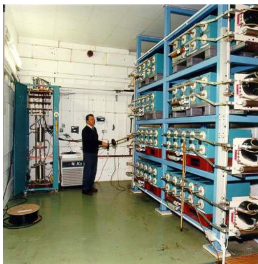
Figure 66. The CLF's Ray Wyatt inside the VULCAN capacitor bank showing ignitrons in the left cabinet and HVR resistors in the main circuit. (Picture courtesy of STFC.)
