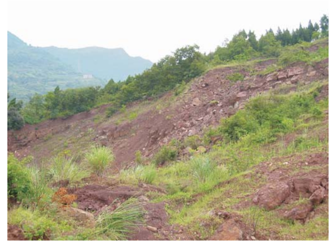
Fig. 11. Site of the excavation of shale as raw materials for brick fabrication.
