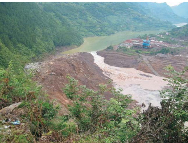
Fig. 8. A channelized diversion excavated for prevention of up-stream flooding and possible damage downstream.
