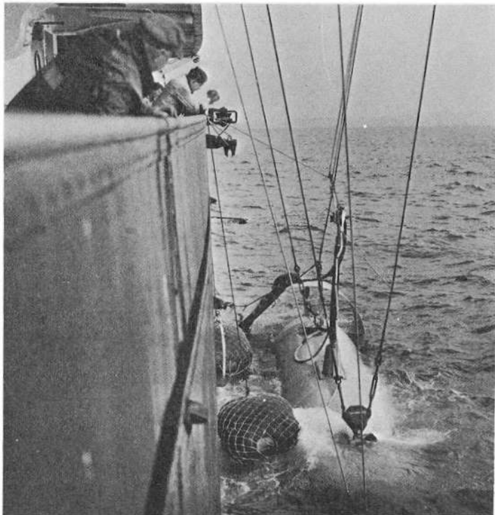
FIG. 7. — The vehicle being deballasted alongside Discovery before being hoisted aboard.
