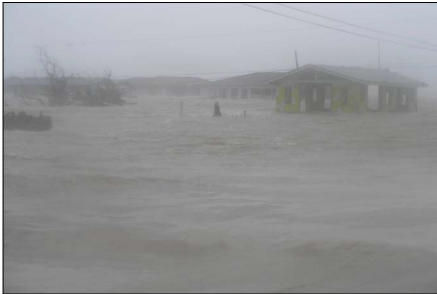
Picture B.32 – Hurricane Wilma Damage on the Island of Grand Bahama, The Bahamas (Source: NEMA, 2004)
