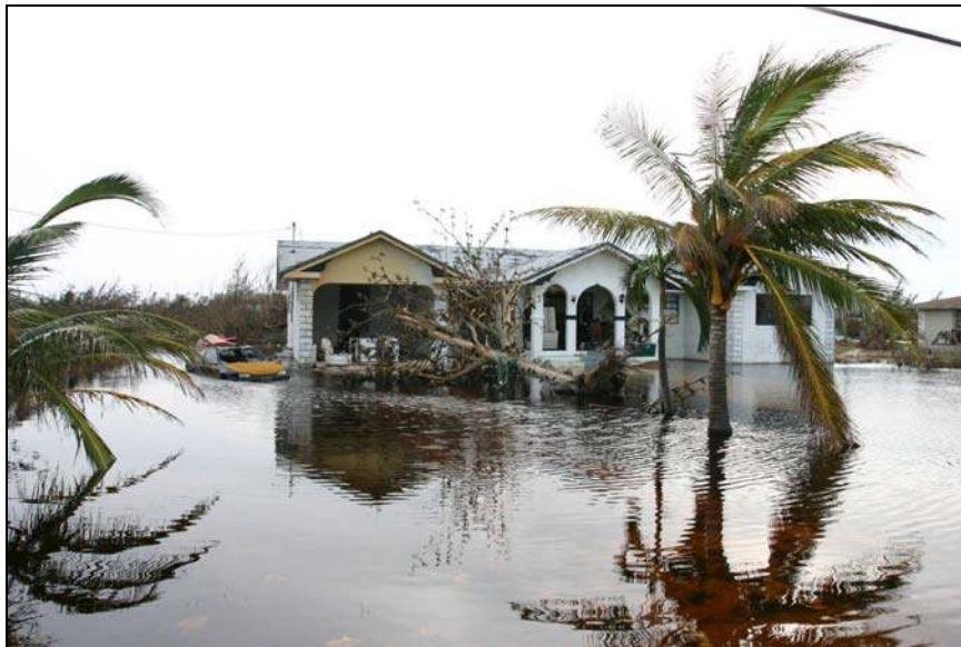
Picture B.14 – Hurricane Frances Damage on the Island of Grand Bahama, The Bahamas (Source: NEMA, 2004)
