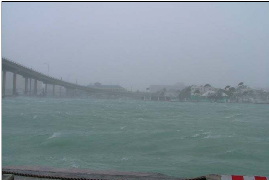
Picture B.22 – Hurricane Frances Damage on the Island of New Providence, The Bahamas (Source: Erin Hughey, 2004)
