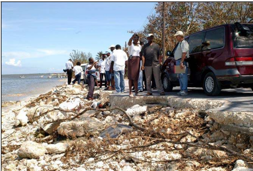
Picture B.20 – Hurricane Frances Damage on the Island of Andros, The Bahamas (Source: NEMA, 2004)
