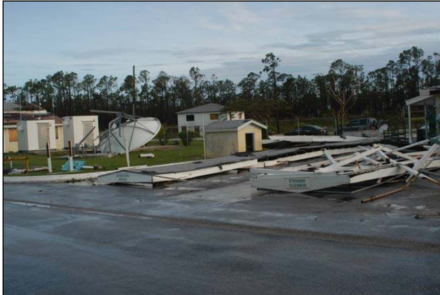
Picture B.24 – Hurricane Jeanne Damage on Treasure Cay, The Bahamas (Source: NEMA, 2004)
