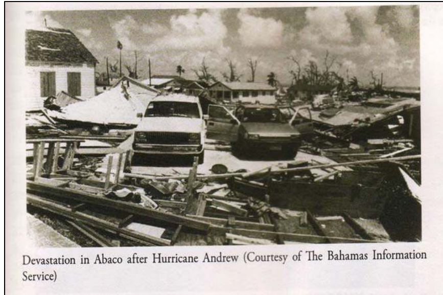
Picture B.2 – Hurricane Andrew Damage on the Island of Abaco, The Bahamas. (Source: The Bahamas Information Service published in Neely 2006)
