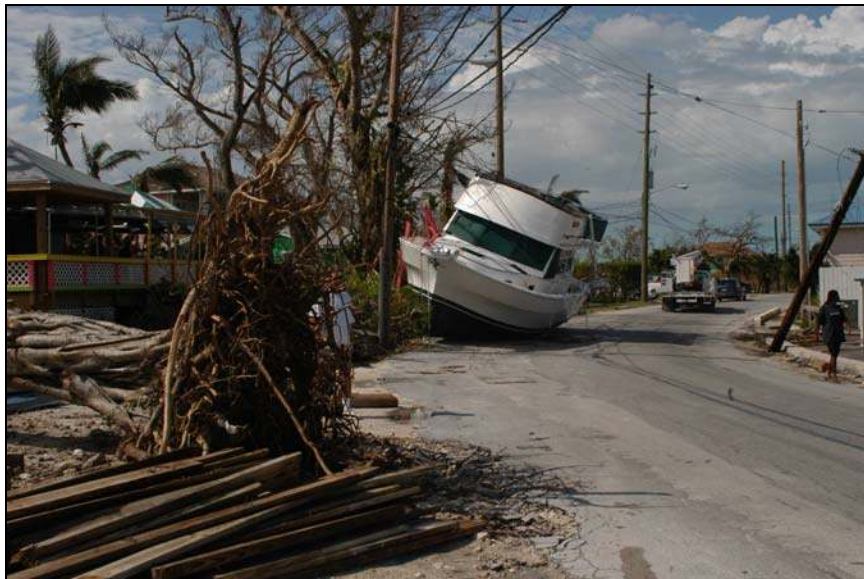
Picture B.25 – Hurricane Jeanne Damage, Abaco (Source: NEMA, 2004)
