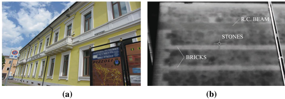
Fig. 4 The Pizzoli town hall building. a View of the façade, highlighting the elongated shape and the regular arrangements of openings on the perimeter walls. b Infrared thermography of a lateral perimeter wall, revealing the masonry typology made up of simple stones with brick courses. A reinforced concrete edge beam is visible at the floor diaphragm level
