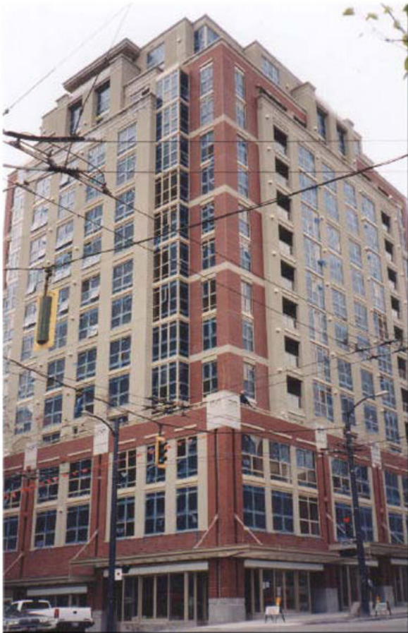
Figure 10. Photograph of Heritage Court Tower (HCT) building.
