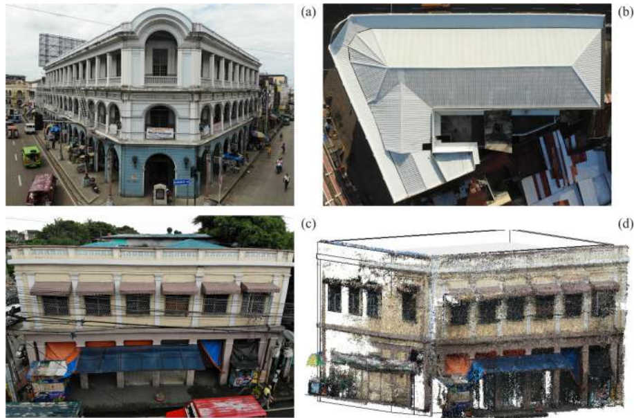
Figure 6. Use of new technologies for the survey of the Iloilo City CH assets: Villanueva building front façade (a), and roof (b) by drone; Villanueva building 6 front façade (c) and point cloud (d) by drone and photogrammetry respectively.
