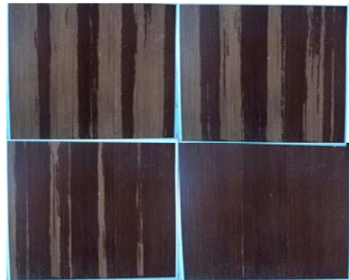
Figure 6. Watered area of cooling pad.
