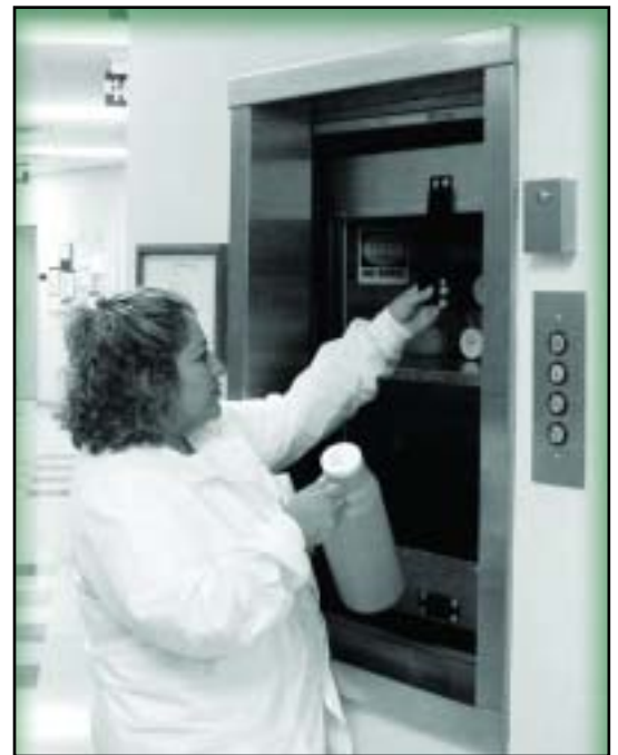
Image 6_Dumb waiter used to transport samples from the outpatient phlebotomy area to the central specimen processing area directly below.
