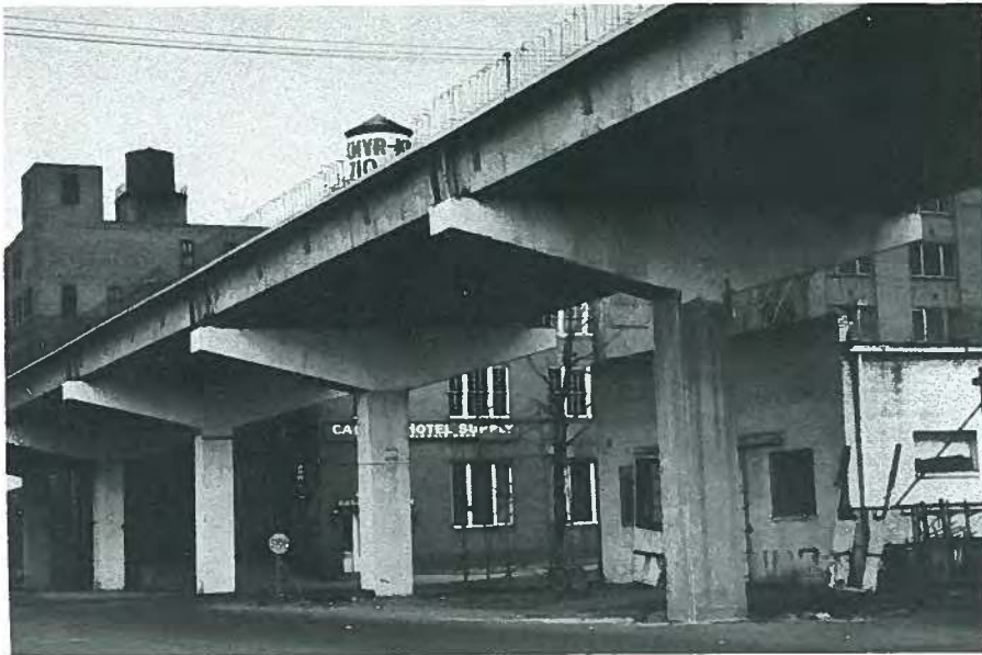
Fig. 23. In 1956, precast single-tee sections for a viaduct were made at Prestressed Concrete of Colorado's second pretensioning plant and transported to the site.
