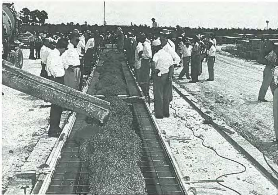
Fig. 29. Demonstrating the production of a 14-in. (356 mm) deep by 4-ft. (1.2 m) wide double-tee at R. H. Wright & Co., Fort Lauderdale, Florida. Note that this form used a steel liner for the stems only. The remainder of the form was concrete.
