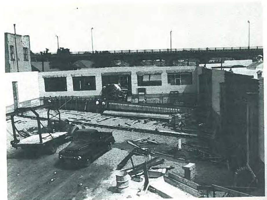
Fig. 22. Post-tensioned beams were cast on site at the Star Bakery because of the limitations of existing transportation equipment.
