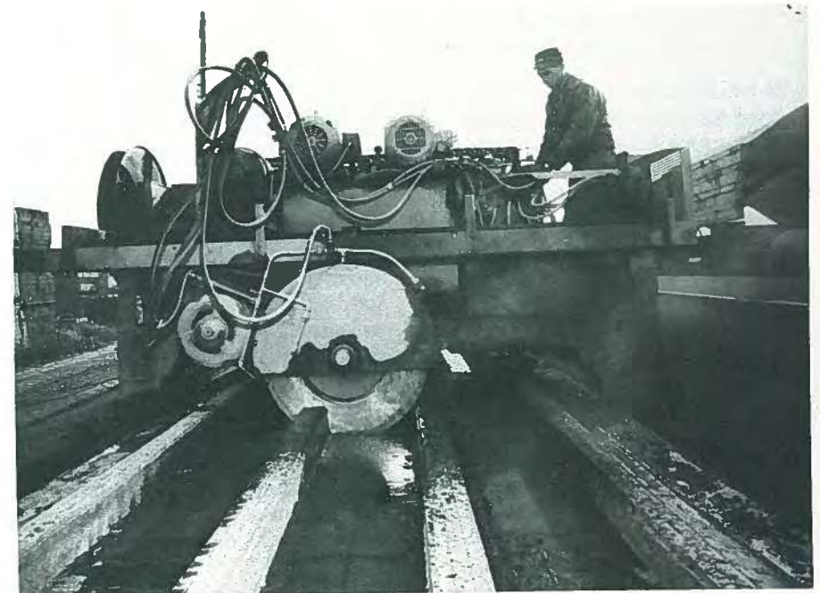
Fig. 26. After the concrete set, the Quadeck was cut to size by a saw attached to the machine.
