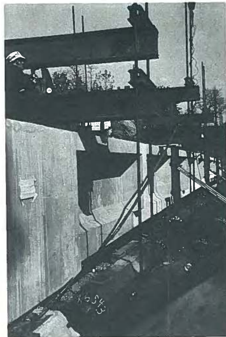
Fig. 7. Looking east, showing loading arrangement on Walnut Lane test girder. Steel ingots are in foreground.
