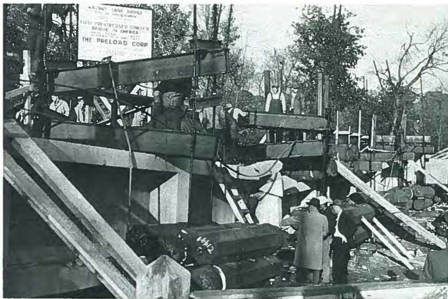
Fig. 11. General view immediately after destruction of Walnut Lane test girder. Failure occurred at 3:00 p.m., October 27, 1949.
