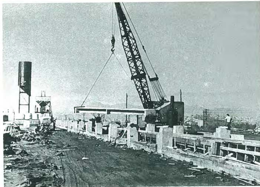
Fig. 11. A single-tee slab is lifted off the bed ready for transport to the Spitzer Electric Company.
