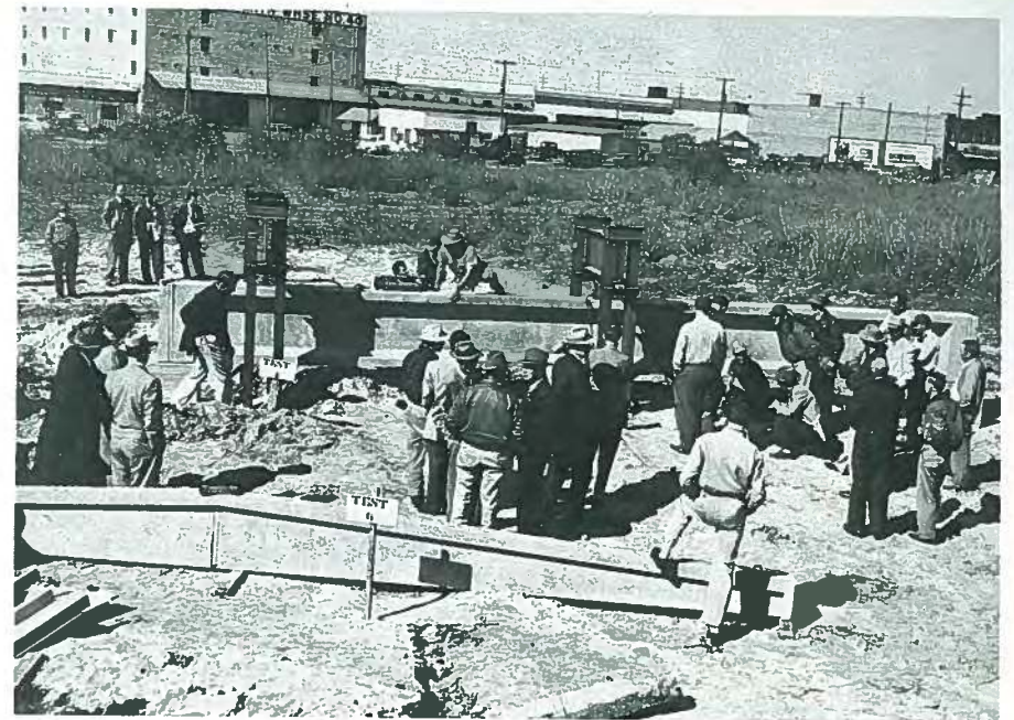
Fig. 26. Demonstration test of prestressed I-beam at Cone Brothers Construction Co., Tampa, Florida. In foreground is a variable depth tee-joint. Courtesy: Paul Zia.
