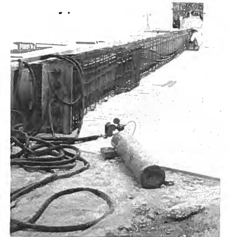
Fig. 19. Forms with inflatable rubber voids.
