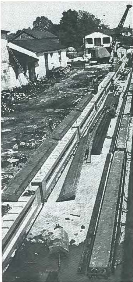
Fig. 12. Pretensioned bonded "I" section girders at casting plant in New Orleans for the production of girders for Loyola University's stadium about 1953.
