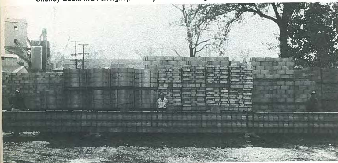
Fig. 17. Continuity test at Breeko Plant. On the left is Lloyd Markham, at center Charley Scott. Man on right probably carried loading blocks. Taken in August 1952.
