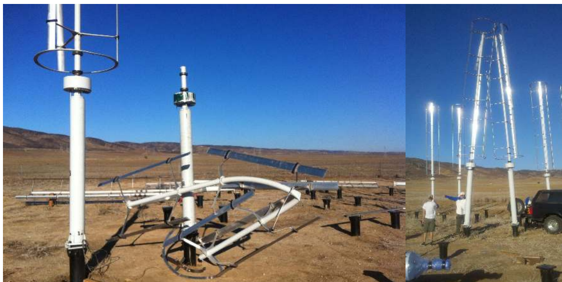
FIGURE 4. Examples of VAWT structural failures at the Caltech Field Laboratory for Optimized Wind Energy (FLOWE).
