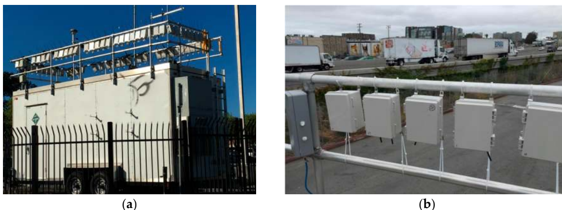
Figure A1. (a) Over 60 ABCDs hung from the roof railing of the Bay Area Air Quality Management District roadside monitoring station in Oakland, California; (b) Close up view of ABCDs deployed at the monitoring station, with California Highway 880 in the background.
