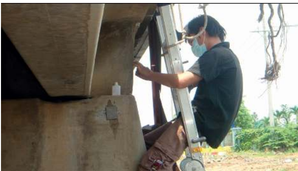
FIGURE 12: Measuring vibrating signals at Ben Noc bridge.
