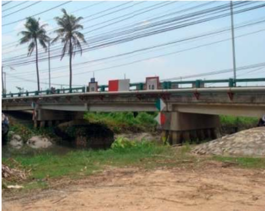
FIGURE 7: Picture of Ben Noc bridge in practice.
