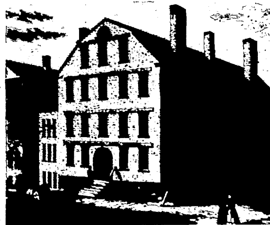
Gambrel roof, The Old Jail.
