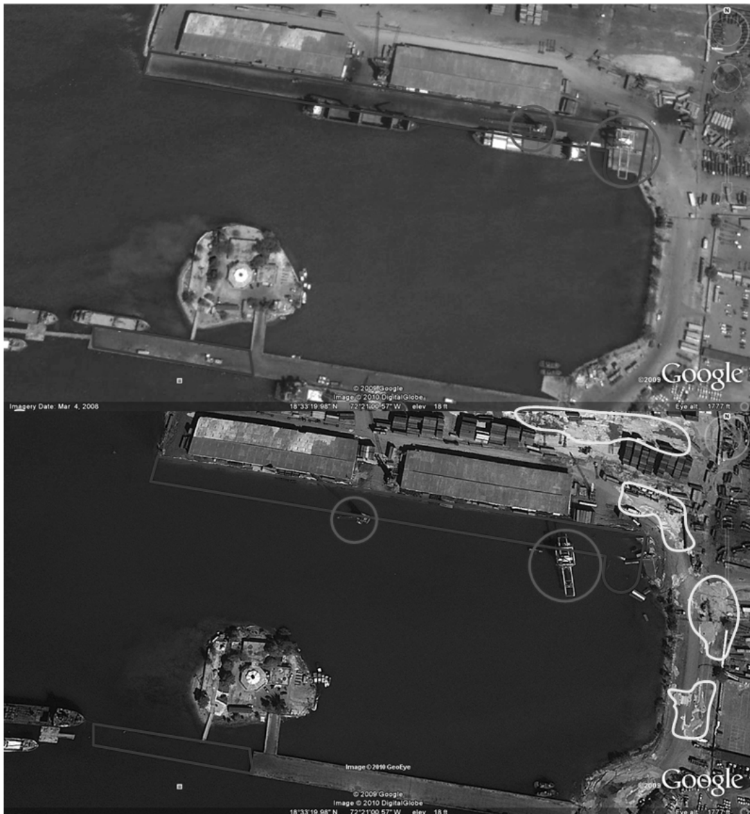
Figure 1.5 Satellite image of Port de Port-au-Prince before and after the 2010 Haiti earthquake showing the collapsed wharf, submerged cranes and sand boils (Google [3])
