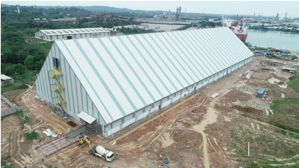
Figure 12. The new fertiliser warehouse building.
