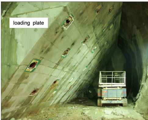
Fig. 2. Chamber tunnel and loading plate(Yi Sun-sin bridge)
