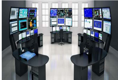
Figure 1: Control room setup https://www.winsted.com/markets/oil-gas/
