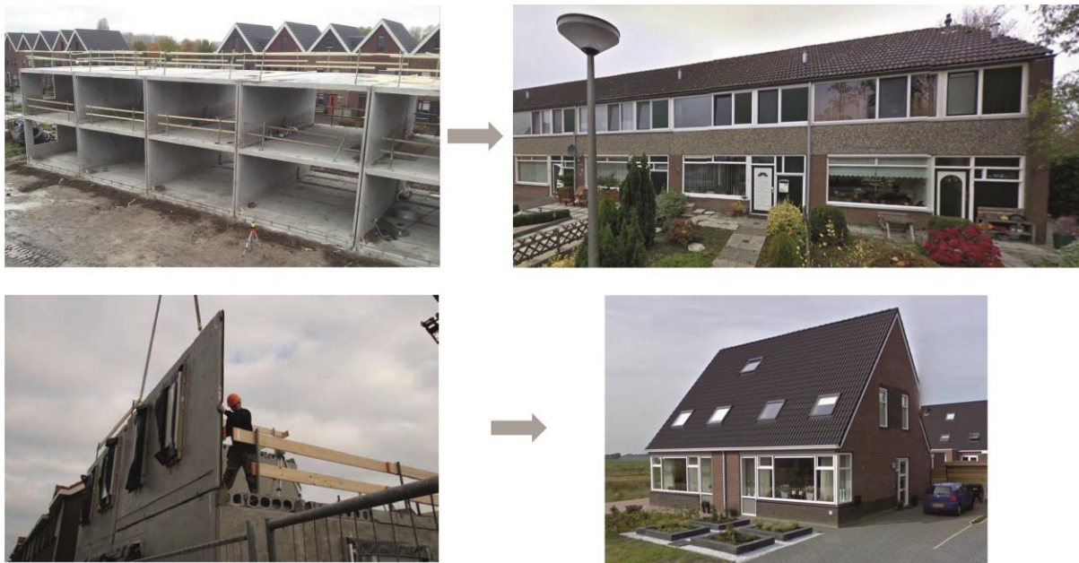
331 Figure 5. Examples of reinforced concrete construction (with masonry cladding) in the Groningen 332 region: cast-in-place (above), precast (below) 333
