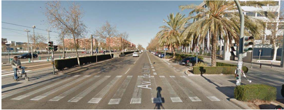
Figure 2- Photograph of Avenida de los Naranjos: it has a section of 70 meters, with 4 traffic lanes in each direction and a tram lane in the middle. Source: Google Street View (accessed on 20 th October 2014).
