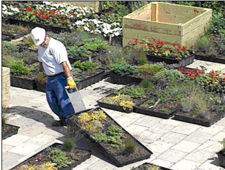
Figure 17: Modular green roof systems (Weston Solutions, Inc., 2009)
