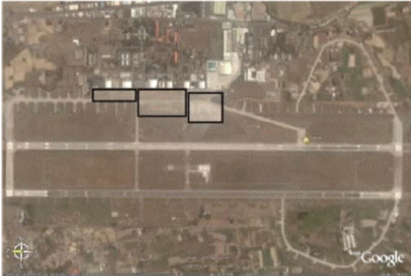
Figure 3.9 Aircraft Parking Ramps on Tainan Air Base
