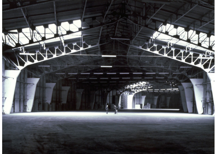
The cavernous Palace of Fine arts building before the Exploratorium moved in.
