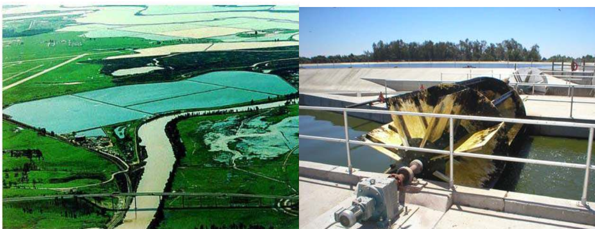
Figure 2.5 and Figure 2.6 Municipal wastewater treatment facilities.
