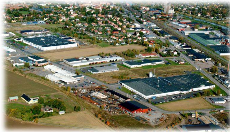
Daloc Ltd. is on the left: Daloc Trädörrar Ltd. is on the right. Photo from 2005.
