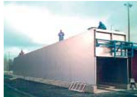
Figure 6. Stainless steel sandwich panels made of austenitic stainless steel grade 1.4301 (AISI 304) used in the wood drying tunnel. (Photo: Kennotech Oy)
