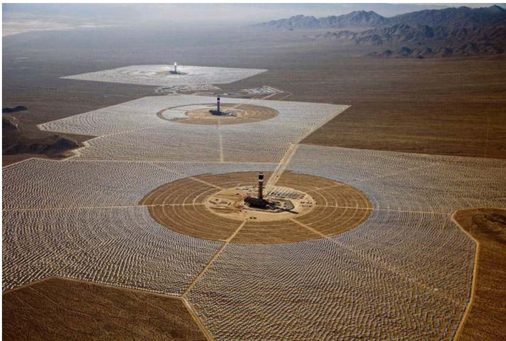
Figure 41. Ivanpah, world's largest solar thermal power plant, uses dry cooling technology
