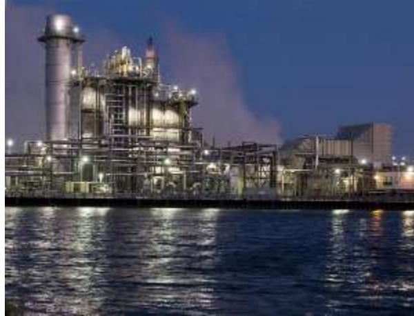
Figure 19 ExxonMobil's Beaumont Refinery in Beaumont, Texas operates a 470-megawatt CHP system that achieves an operating efficiency of 88%
