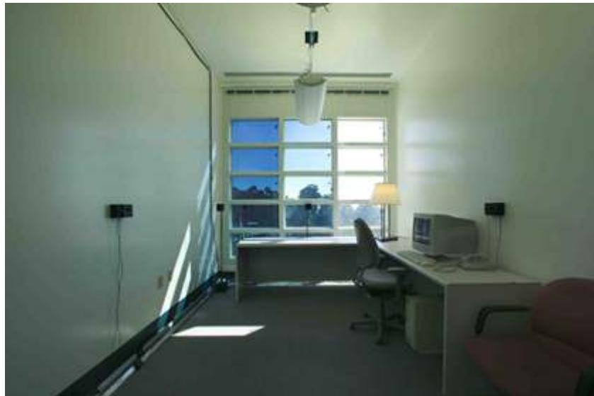
Figure 8. Electrochromic windows, Source: LBNL
