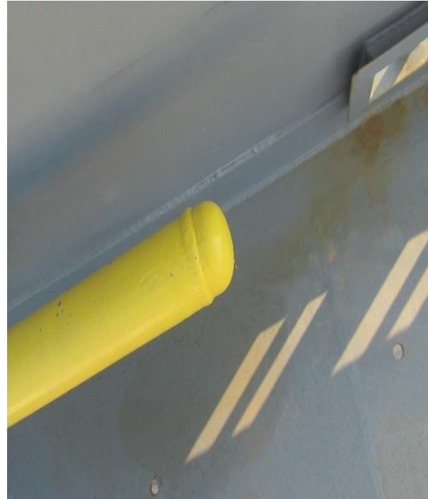
Fig. 59: Foam Ring Main with End Cap
