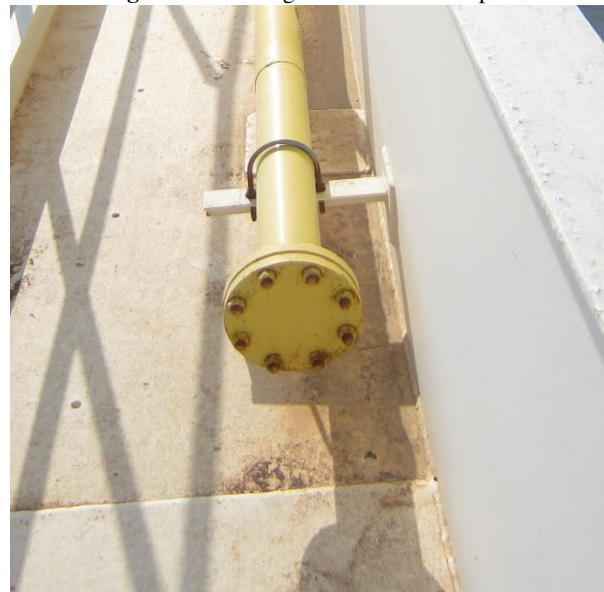
Fig. 60: Foam Ring Main with Flanged End
