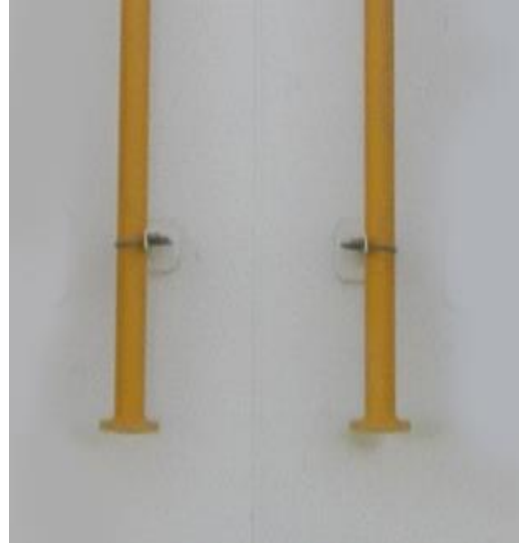
Fig. 42: Foam System with No Fire Department Connections
