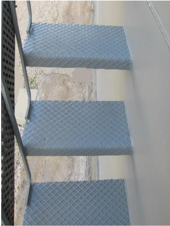
Fig. 17: Spiral Stairway with Steps Attached to Tank Shell
