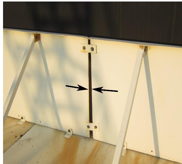
Fig. 4: Foam Dam Fastening Using Nuts and Bolts
