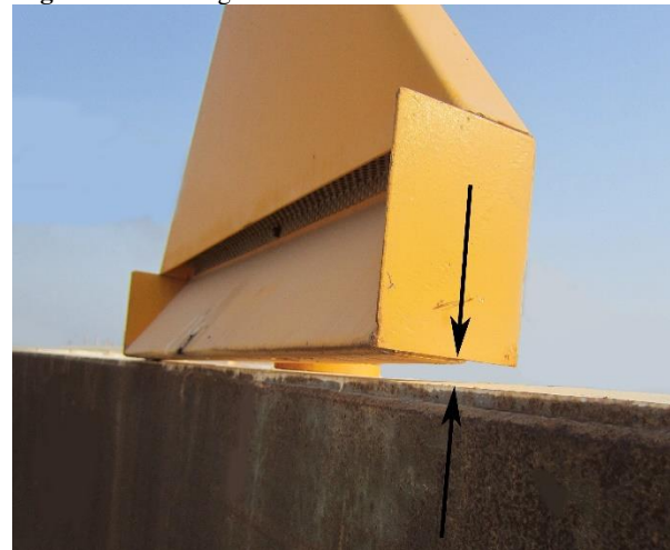
Fig. 46: Foam Pourer Not Fixed to Top Angle
