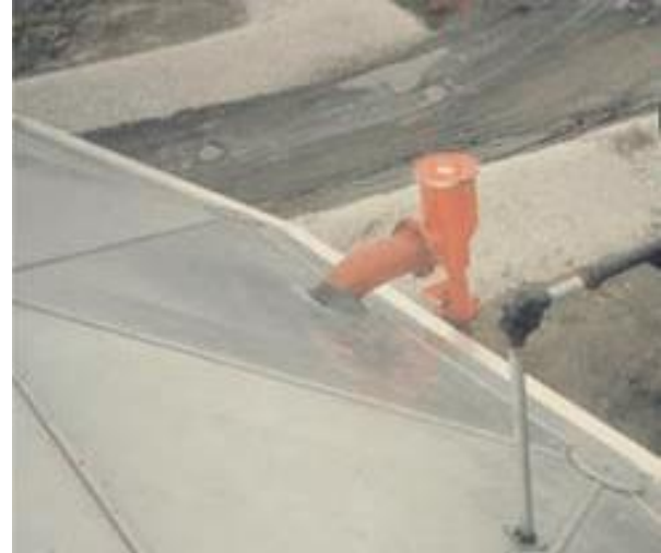
Fig 50: Installation of Foam Pouwer on the Roof of Fixed Roof Tanks
