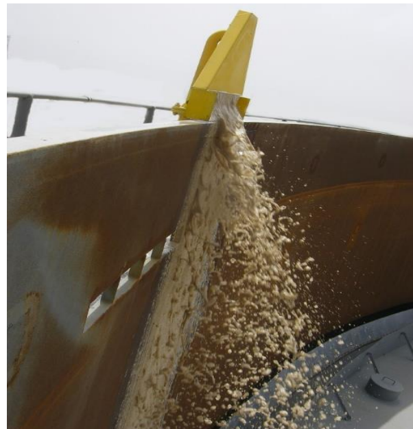
Fig. 43: Throwing of Foam Stream by Foam Pourer
