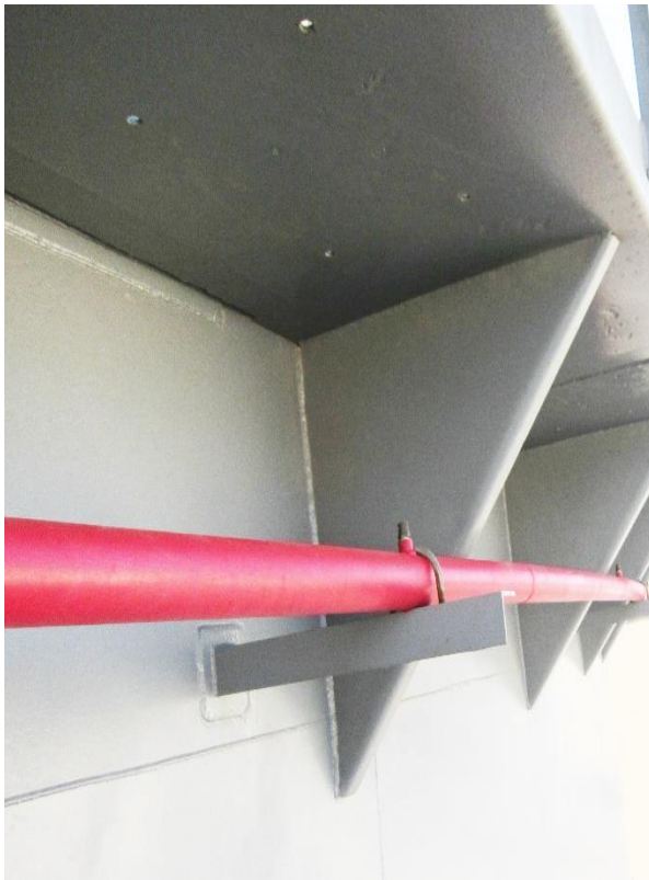
Fig. 13: Water Curtain Blockage by Triangular Support Members
