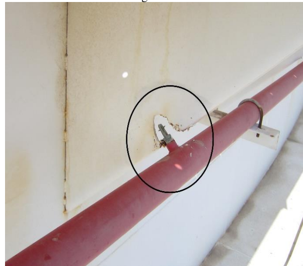
Fig. 26: Cutting Wind Girder Support to Allow Installation of Spray Nozzle
