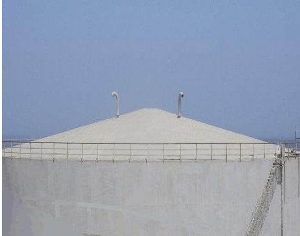
Fig. 32: Fixed Roof Tank with No Roof Protection
