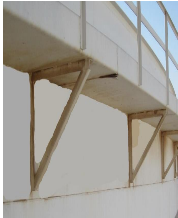
Fig. 14: Slender Support Member for Walkway
