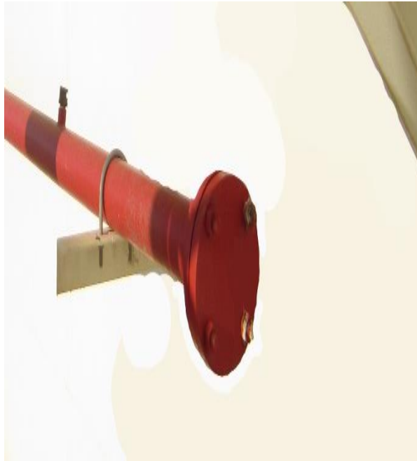
Fig. 37: Ring Main with Flanged End
