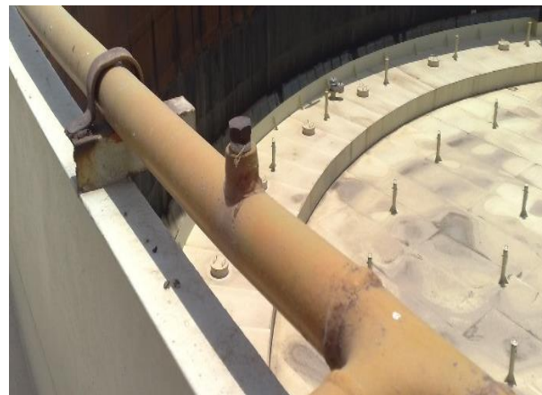
Fig. 56: Tap for Pressure Gauge
