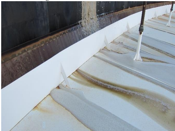
Fig. 2: Excessive Foam Drainage from under the Foam Dam Due to Non-standard Slot Size
